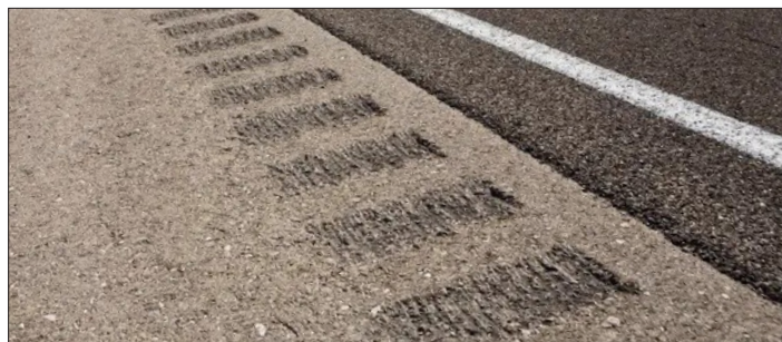
Figure 3. Short milled rumble strips adaptable to airport use. (Photo courtesy of the U.S. Department of Transportation Federal Highway Administration)
