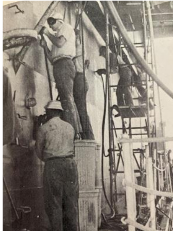
Sailors use stacked trashcans as a makeshift work platform (Photo courtesy of Fathom magazine, 1969)
