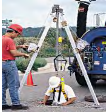
Tripod used for safe entry
