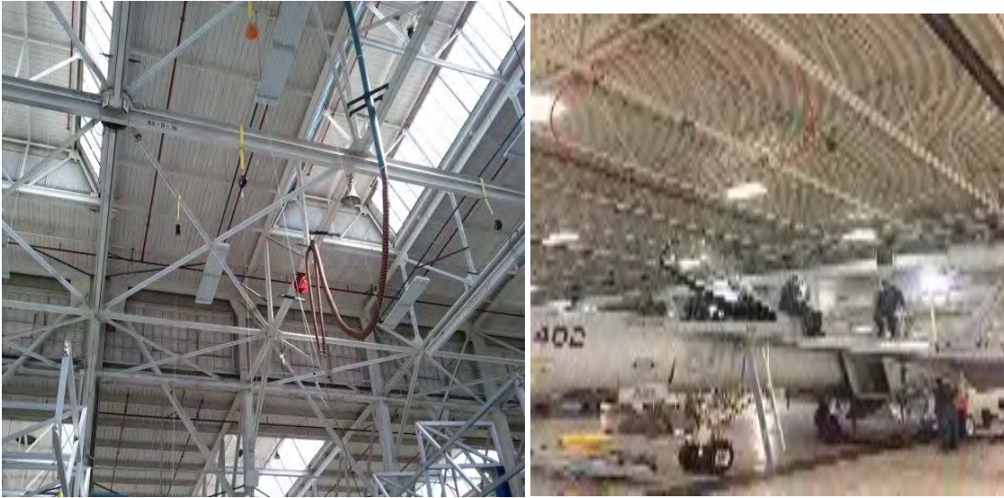
Overhead Beam Strap with Self Retracting Lanyard
