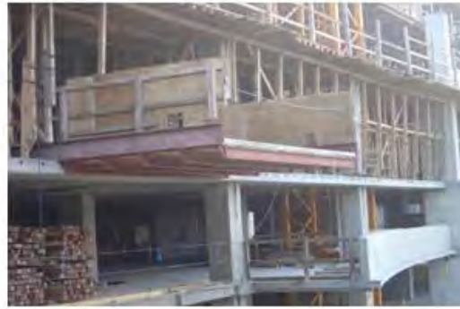
Loading Platform w/Removable Chain at point of access, however Mid Rail is also Required
