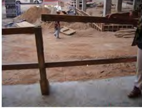
Removable Guardrail at second Floor
