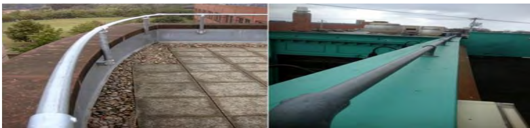
Above, solutions using additional railing to make parapets comply with OSHA 42-inch height requirement.
