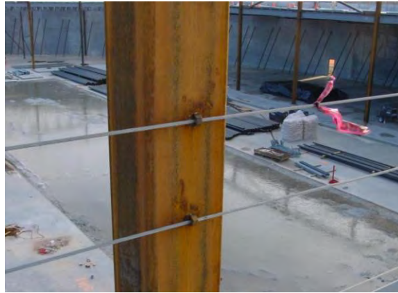
Steel Cable Guardrail
