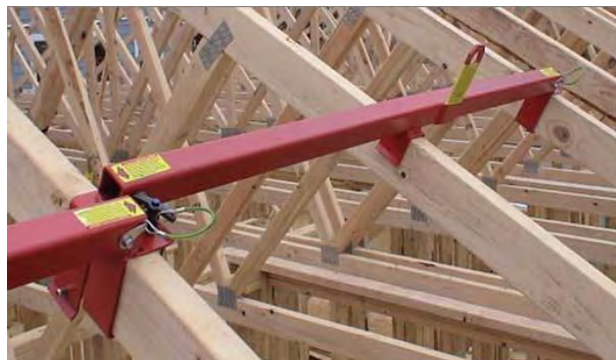
Anchorage connector for wood construction that spreads the fall forces on more than one rafter
