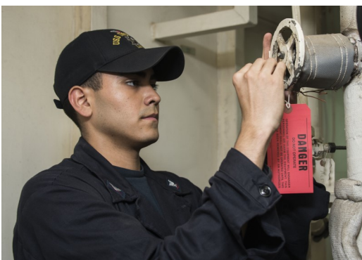
Engineman 3rd Class Adam Salcedo hangs a danger tag for maintenance in the laundry room aboard the Wasp-class amphibious assault ship USS Iwo Jima (LHD 7) . (U.S. Navy photo by Mass Communication Specialist 3rd Class Dominick A. Cremeans/Released)
