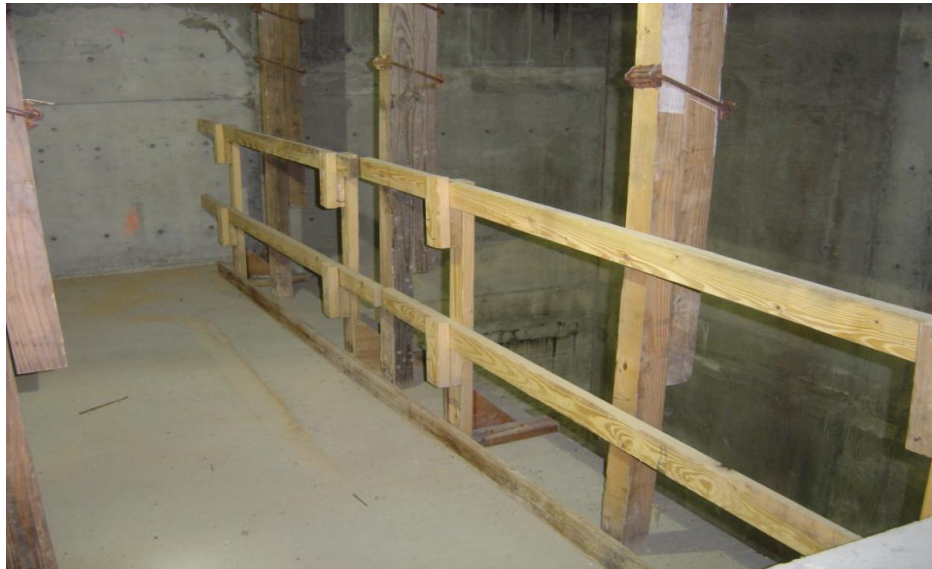
Temporary Guardrail
