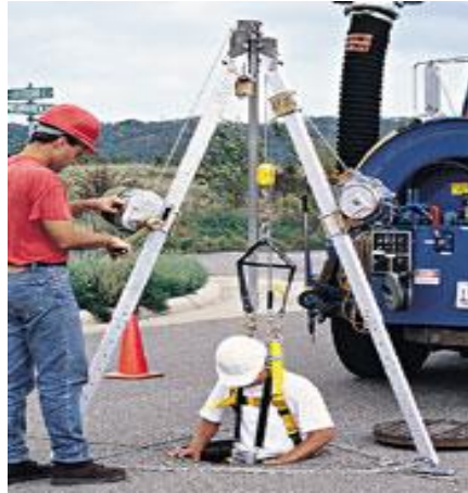
Tripod used for safe entry
