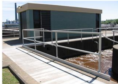
Permanent Pipe Railings
