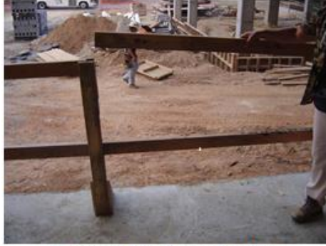
Removable Guardrail at second Floor
