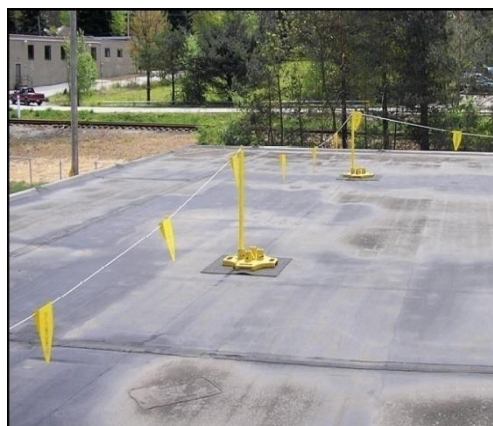
Warning Line System
