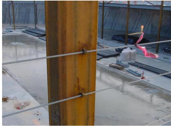
Steel Cable Guardrail
