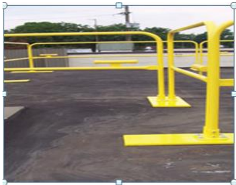
Permanent Pipe Railings
